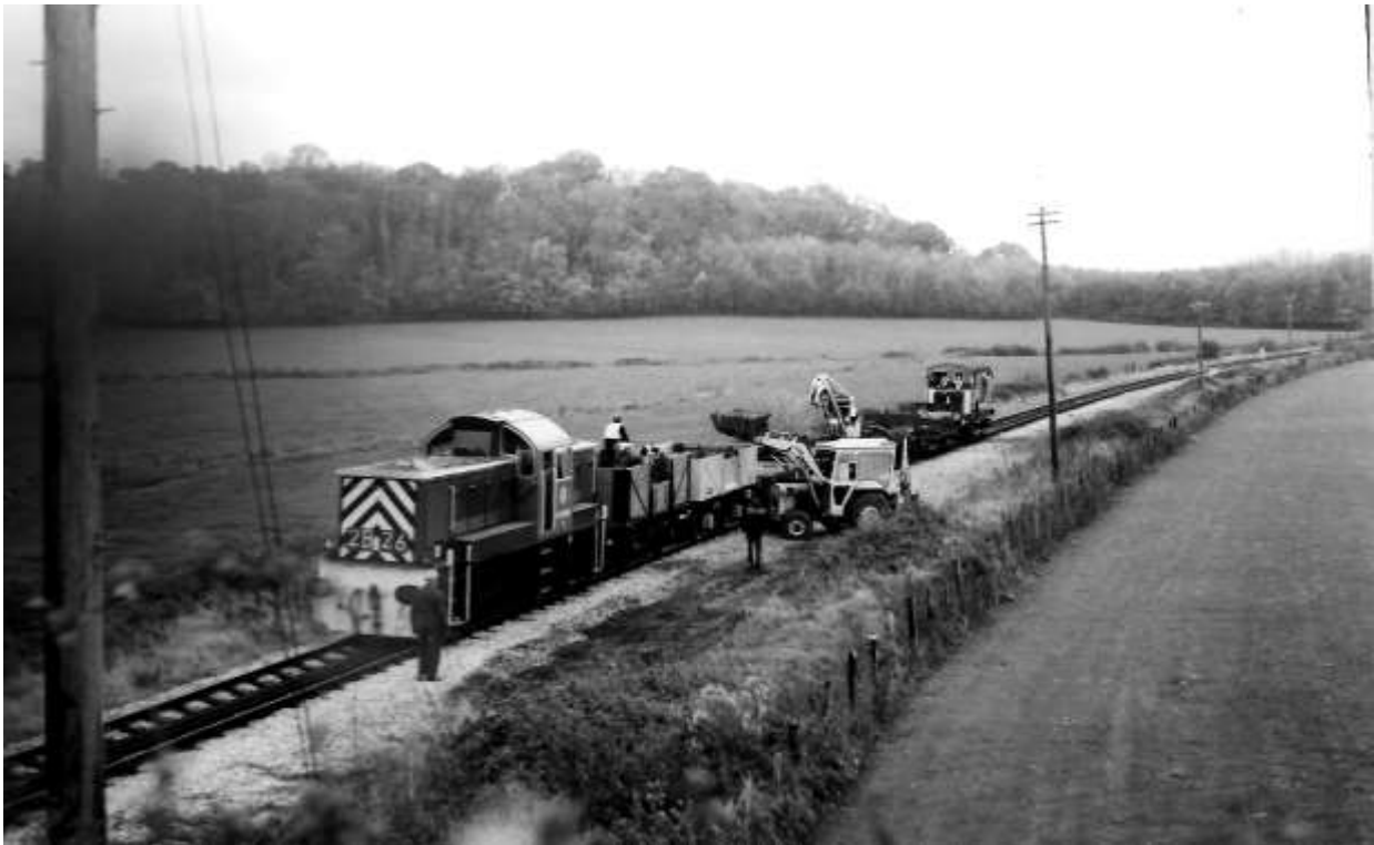
Working engineer's train Photo ( PJ Hembry )
