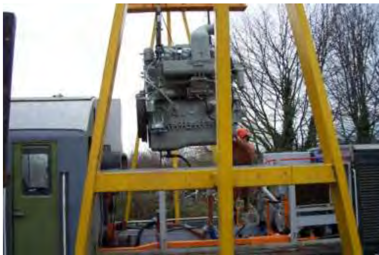
Fitting of overhauled engine Photo (I Robbins)
